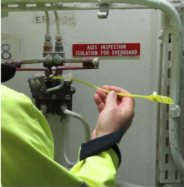
Figure 11 Seal being applied to overboard disposal valve of food grinder
