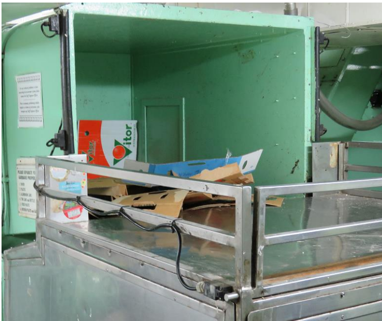
Figure 9 Cardboard being fed into on-board incinerator
